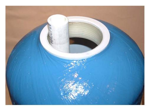
Step 6: Place the funnel into the filter tank as shown below, and slowly pour the gravel and carbon into the filter tank. Caution: If you purchased a filter that came with a bag containing gravel, you must add the gravel first before the carbon.
