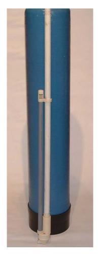
Step 4: Make sure you place the softener tank shown above where you want to connect it to your water line because it will be heavy a difficult to move after the resin is added. Make sure you install your softener in line before your hot water heater to insure that you have full benefit of the softener system.
