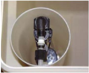
On the Fleck 5600 there is a side connection where you will connect the drain line also. There is a hose barb fitting provided to make this connection. This connection is just to the right of where you just connected the brine tubing line.
