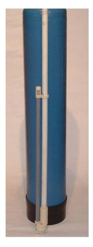
Step 4: Make sure you place the filter tank shown above where you want to connect it to your water line because it will be heavy a difficult to move after the filter media and gravel are added. Make sure you install your filter in line before your water softener.
