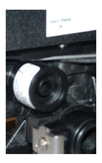
Step 11: The 7000SE control valve head can now be screwed onto the softener tank. Be sure the large O-ring is in place, and lubricated. As you start to screw the control valve onto the tank, make sure the hole in the center of the control valve fits over the riser tube. The control valve should be hand tightened clockwise, snug and tight to eliminate a possible leak.
